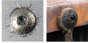
Dome head (Truss)
